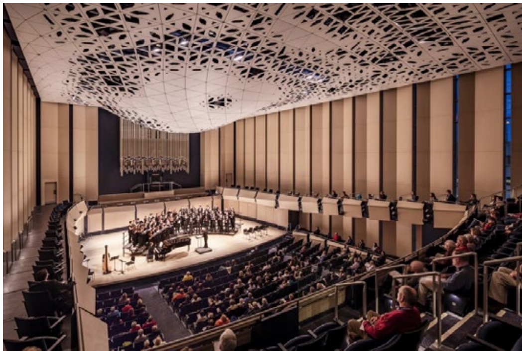
Figure 3.03 The Voxman Music Building's Theatroacoustic Ceiling System uses a carefully designed curved surface to make sure that sound is reflected evenly after bouncing from the stage to the ceiling and back onto the audience. The cut-outs are similarly designed and positioned to absorb sound to prevent echoes and dissonance.
