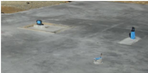
Figure 28: Redundant services in concrete floor can be added during construction for future use. Photo by author.
