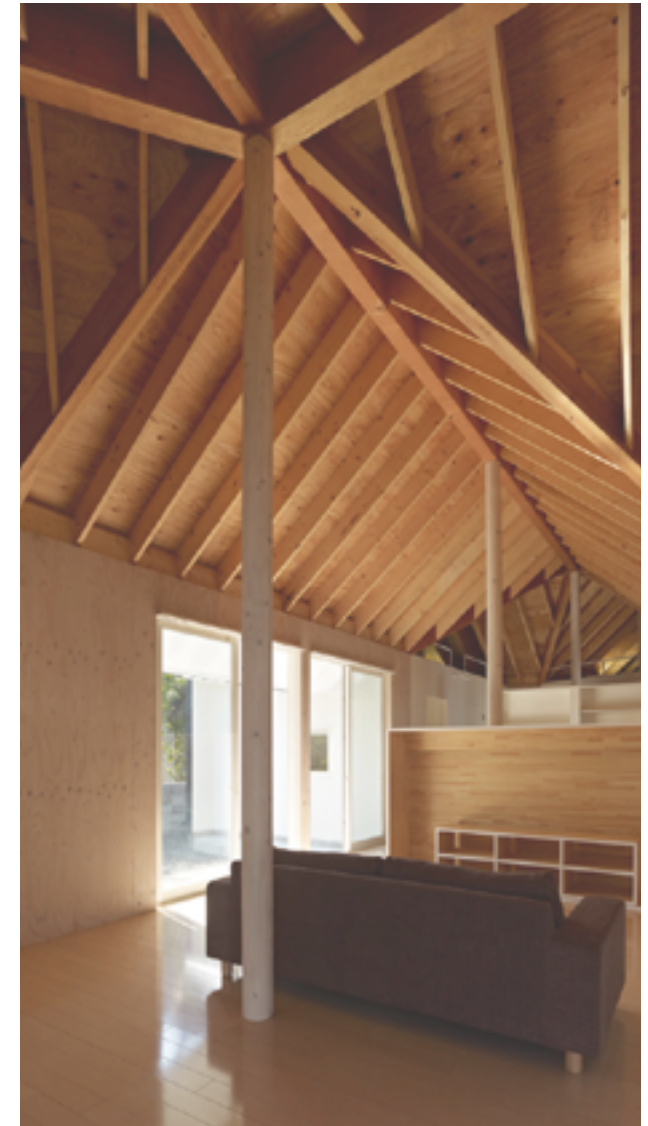
Figure 84: Branch House demonstrates an interesting tactic in legibility. The internal walls are not even touching the roof so they are clearly non-loadbearing.
