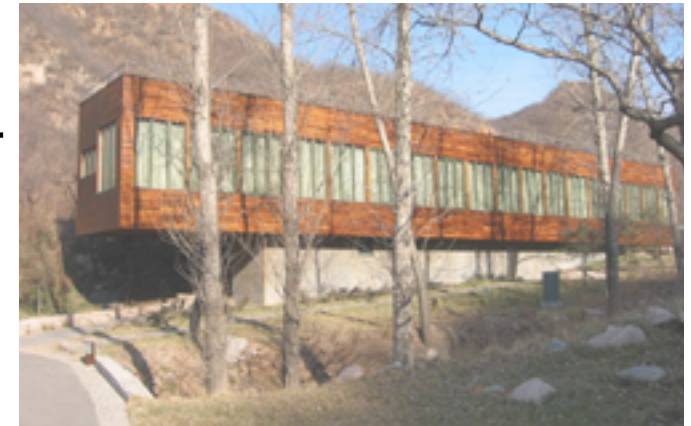
Figure 70: The Suitcase House both sits on the ground plane (ground floor) and is elevated from it (first floor). The elevation above the ground in the first floor allows for several subfloor hatches. The hatches allows bedrooms, kitchens, bathrooms, storage, meditation room, media room and so on to be put away by closing a hatch.
