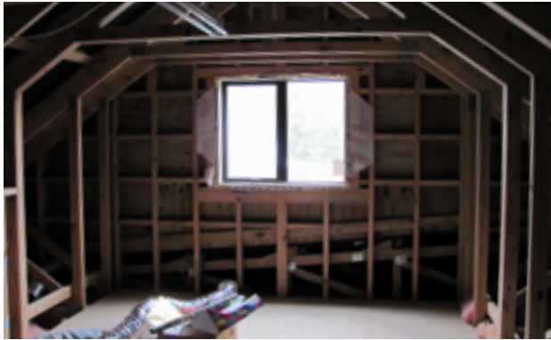
Figure 27: Unfinished attic space designed to be completed at a later date. The shell of the future room is made with attic trusses. The windows, while redundant in the present will provide natural light and ventilation. Photo by author.
