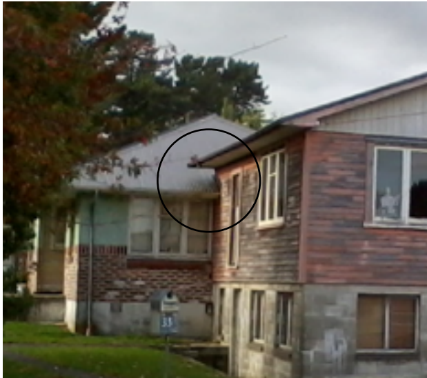
Figure 52: Although the extension of this home will be easy to add-onto with a high stud and gable roof, the connection between the extension and existing gable roof is very poor. Extending onto hipped roofs can result in very messy junctions and internal gutters. Photo by author.
