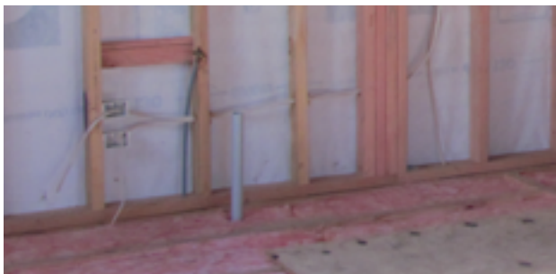
Figure 29: A hole can be cut in the flooring between joists for new services at any location. The ability to crawl under a house makes it easy to add or alter services to houses with a timber subfloor. Photo by author.
