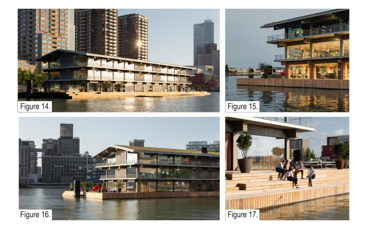
Designing a sustainable, floating office building was a very challenging commission and we approached it in an integrated way. By using the water of the Rijnhaven to cool the building, and by using the roof of the office as a large energy source, the building is truly autarkic – Nanne de Ru (Powerhouse company founder and Architect)
