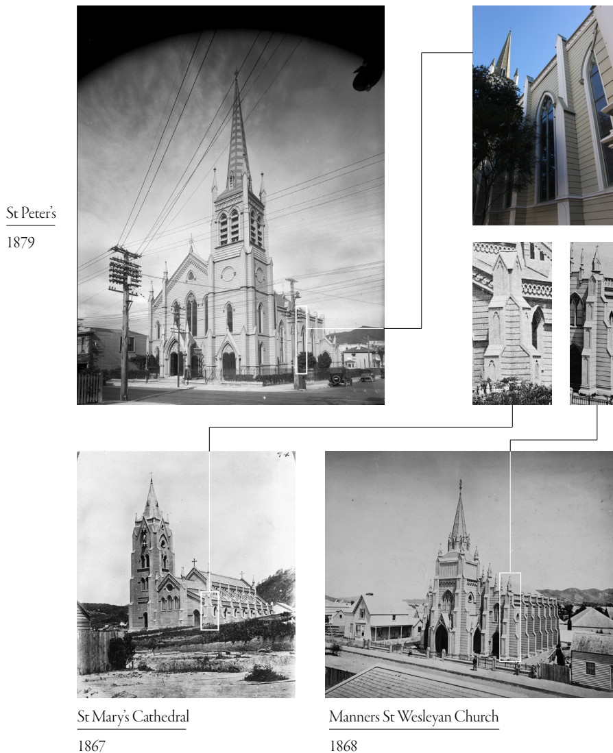
Figure 82. Diagram comparing how the design of the buttresses has changed between the different churches
