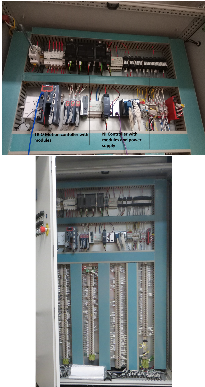
Figure 4.5: Low voltage cabinet of the ss-CAES prototype.
