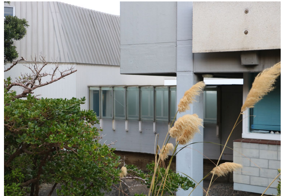
Fig 5.33. Photographs by Author showing connections into the Allen and Brodie buildings that appear to 'slot' in between the structural framework of the building
