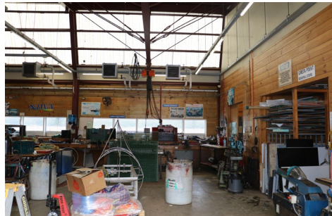
Fig 2.14. Photographs by Author from left to right: view of the interior of the Workshop with equipment everywhere but wooden boards lining the walls are in good condition; structure is all steel with the roof sitting on top and suspended lights
