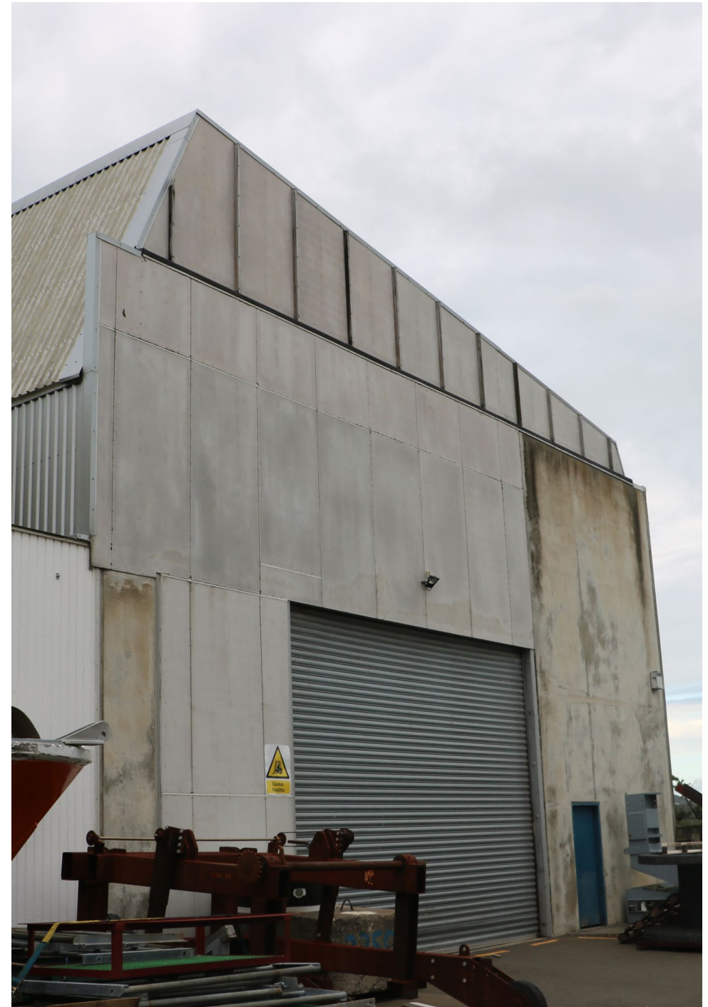
Fig 2.31. Photograph by Author of the exterior of the South Store with large solid concrete panels lining the facade
