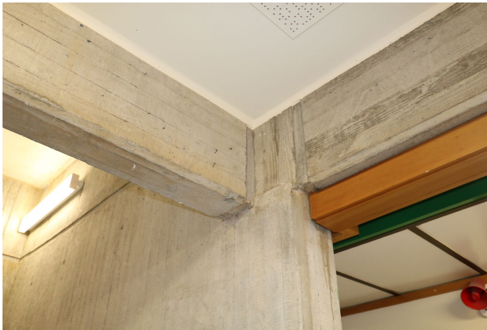
Fig 2.29. Photograph by Author highlighting the exposure of the insitu concrete structure
