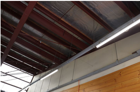
Fig 2.14. Photographs by Author from left to right: view of the interior of the Workshop with equipment everywhere but wooden boards lining the walls are in good condition; structure is all steel with the roof sitting on top and suspended lights
