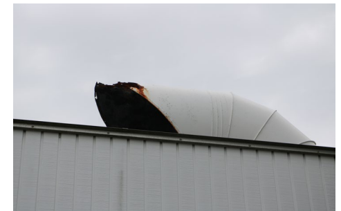
Fig 2.13. Photographs by Author from left to right: the glazed hallway around the outside of the Conference Room that seems to have watertightness issues; a service duct that has been severely affected by the seaside weather conditions
