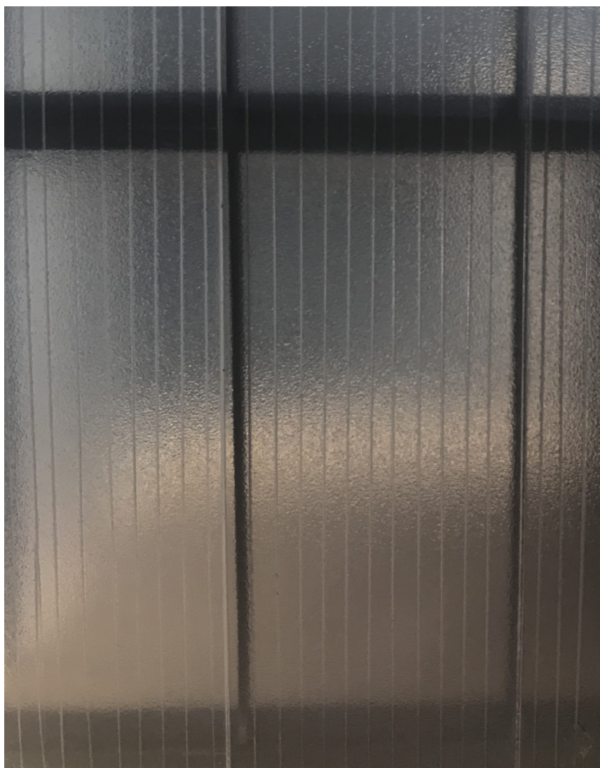
Figure 99./ Photograph of physical model showing the transparency of the polycarbonate cladding which offers different light and privacy qualities.
