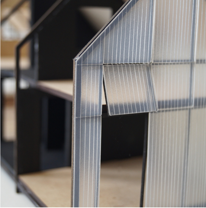
^ Figure 97. / Photograph of physical model exterior materiality and the opportunity to make openings in the polycarb for ventilation.
