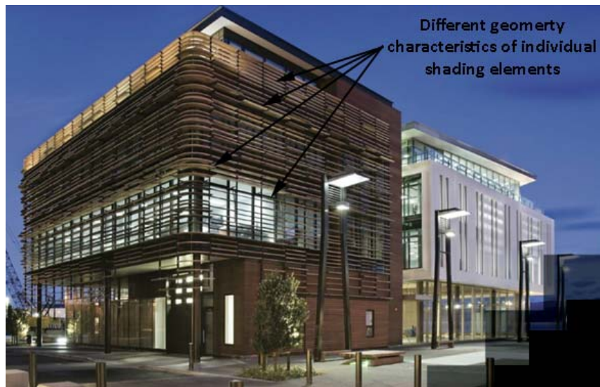
Figure 8-20 : Example Louvre system: Meridian building. Figure adapted from (New Zealand Green Building Council 2013).
