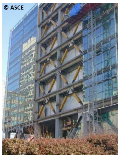
Figure 56. Installation of the braced frames in the Wallace F. Bennett Federal Building (Source: Symans et al., 2008)
