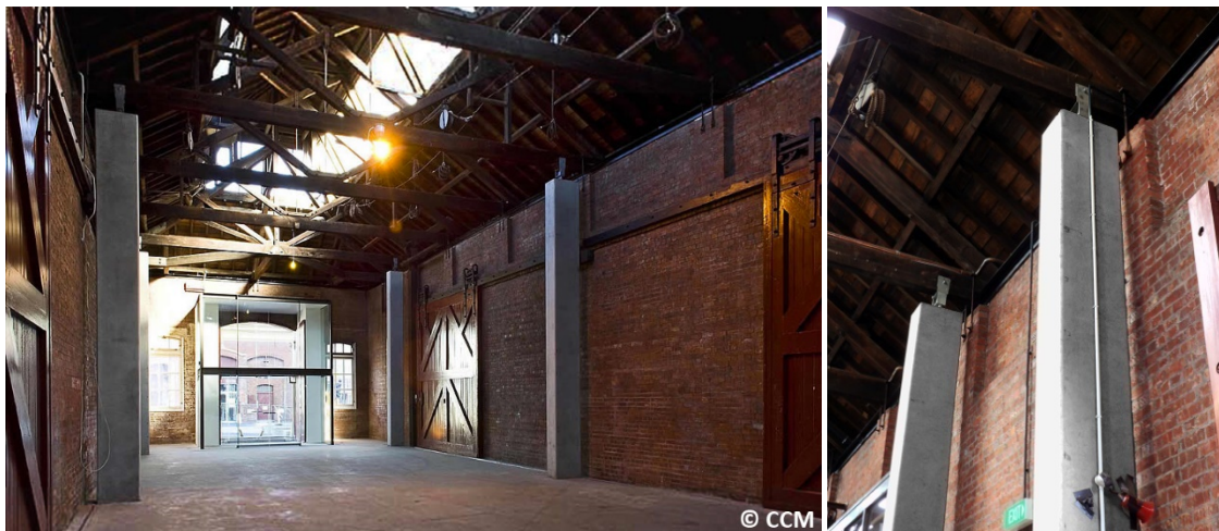
Figure 53. Shed 13 with new concrete columns connected to existing trusses but separated from the URM walls (Sources: Cattanach, 2008, p. 8 and Author)
