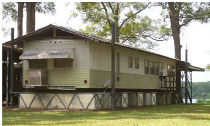
Figure 3.6 Buoyant Foundations, Mississippi, USA. (English 2016)
