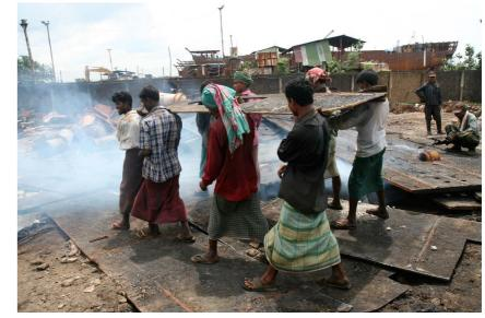
Fig. 3.24 Workers carrying heavy steel plates by hand with minimal footwear
