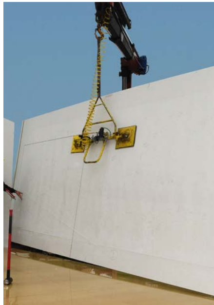
Figure 5.07. Metrapanel wall panels being installed
