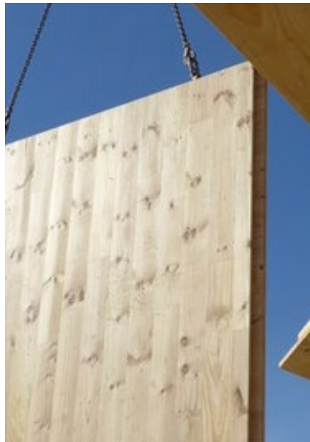
Figure 5.06. Xlam CLT being installed
