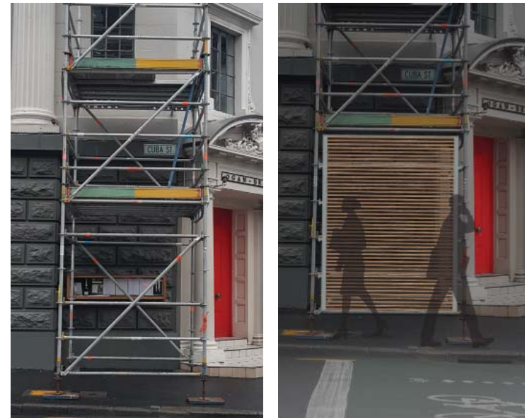
Figure 9.1 : Batten bracing
