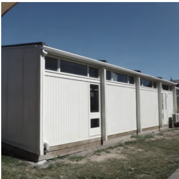
▲ Fig 2.24. CEBUS model classroom these portable units have standard high level windows for cross ventilation. Usually installed on relatively flat sites, the sub-floor is enclosed.
