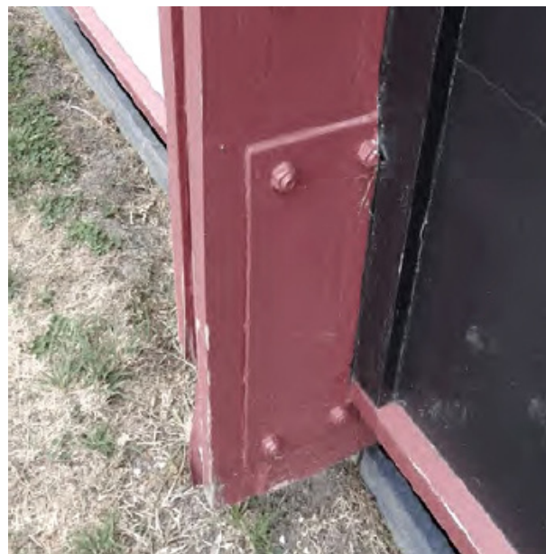
▲ Fig 2.25. CEBUS Typical Module Junction. The junction is expressed, often with a bolted connection for easy disassembly.
