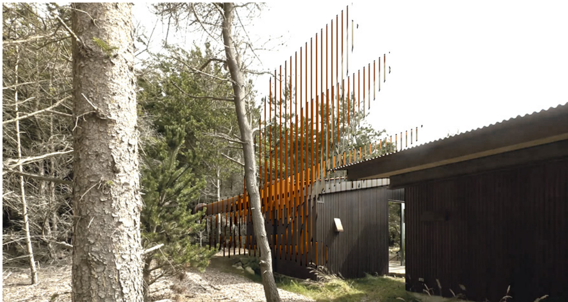
▲ Fig 2.30.Shadowboxx. An actuating roof is used to open an artists studio to the external environment taking advantage of counter-weights to allow for ease of movement
