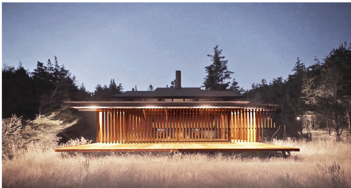
▲ Fig 2.31.Shadowboxx. Actuating facade expands the internal space into the external environment. This transitional method allows for utilisation of the external space dependant on environmental conditions.
