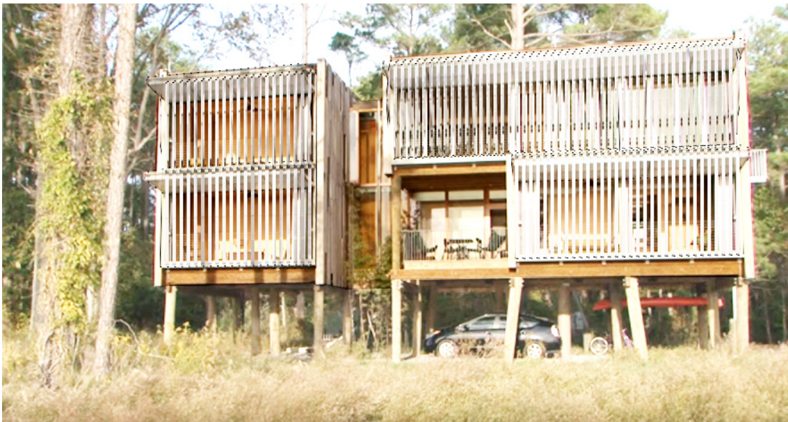
▲ Fig 2.36. Loblolly House. Awnings and a sliding double skin facade allow the internal form to open to the exterior. This undercroft becomes an extension of landscape and awnings shade the internal space.
