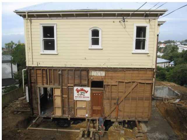
Figure 87: Sarking and Weatherboards – external view.
