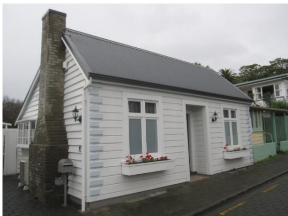
Figure 92: House with Rusticated and Plain Weatherboards, South Street, Nelson
