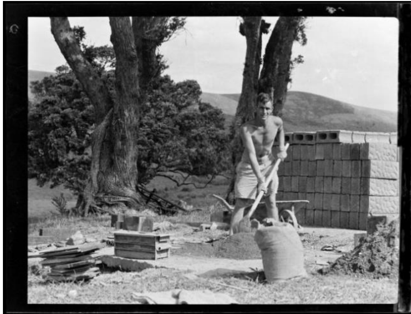
Figure 81: J. Pullman making concrete blocks at Sandy Bay. March 1946
