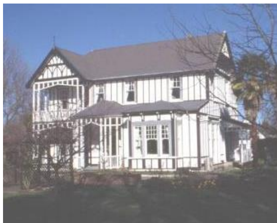
Figure 96: Homebush, Masterton uses precast concrete panels (1890s)
