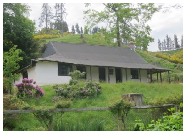
Figure 27: Glens of Tekoa, North Canterbury 1859 (cob, wattle-and-daub internal walls)
