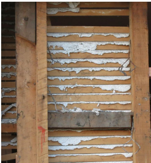
Figure 86: Lath-and-plaster - the view inside the wall
