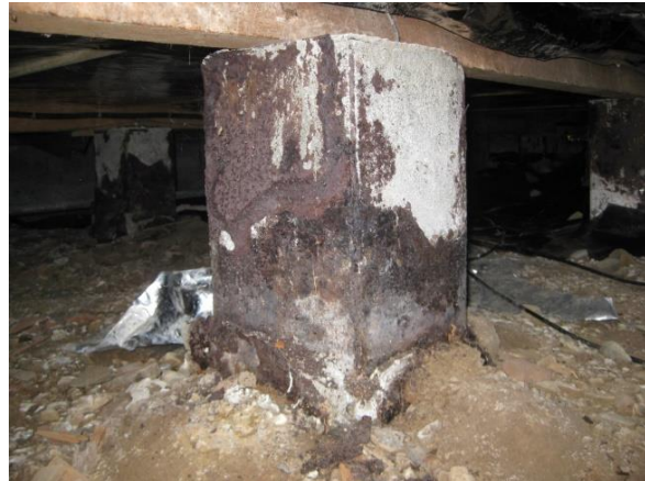
Figure 55: Kerosene Tin filled with concrete used as a house pile
