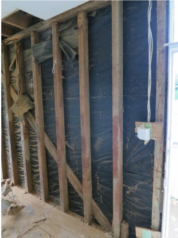
Figure 68: Interior view of platform framing and building paper c1911
