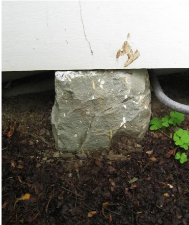
Figure 52: Close view of shaped stone pile and weatherboard at Ranzau (built 1844)
