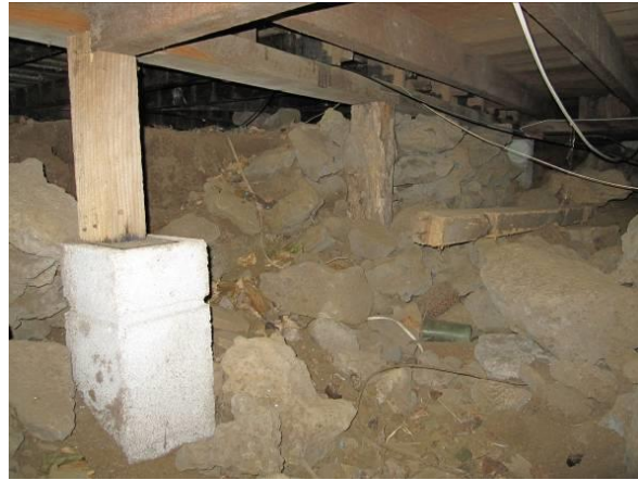
Figure 53: Piles in restored Alberton (built 1863)
