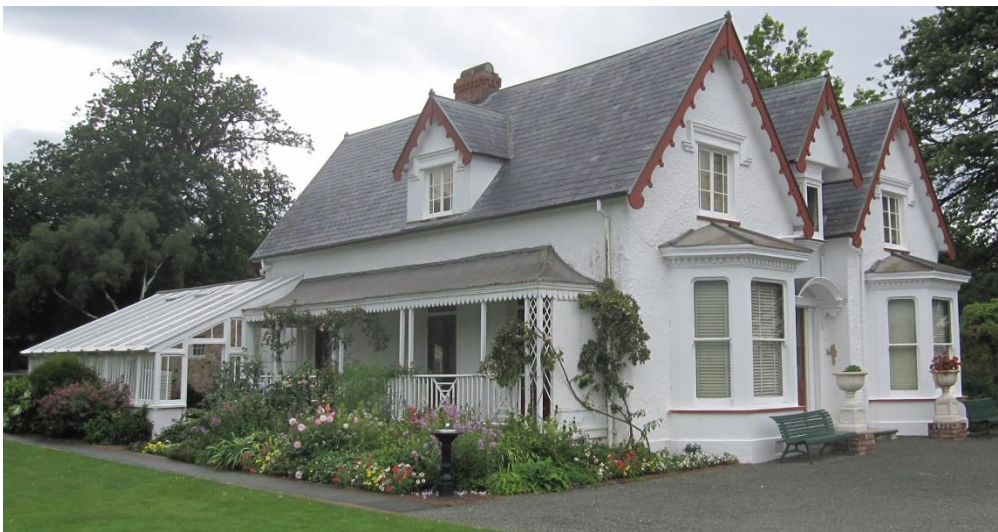
Figure 107: Broadgreen Cob House showing Slate Roof c1855
