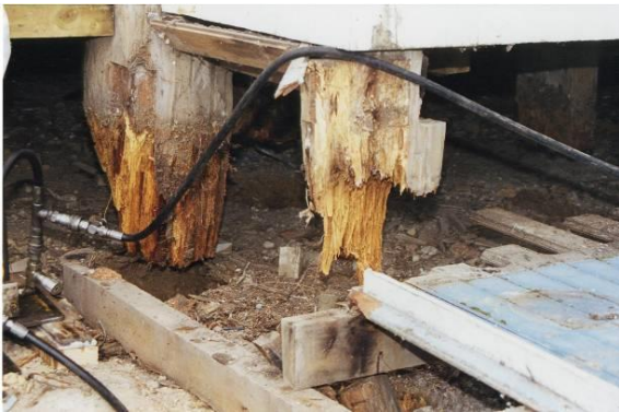
Figure 54: 90 year old Totara piles after house was lifted
