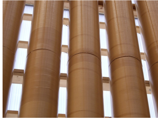
Fig. 23: Detail of Damage to Cardboard Paper Tubes , 2014, photograph. 95
