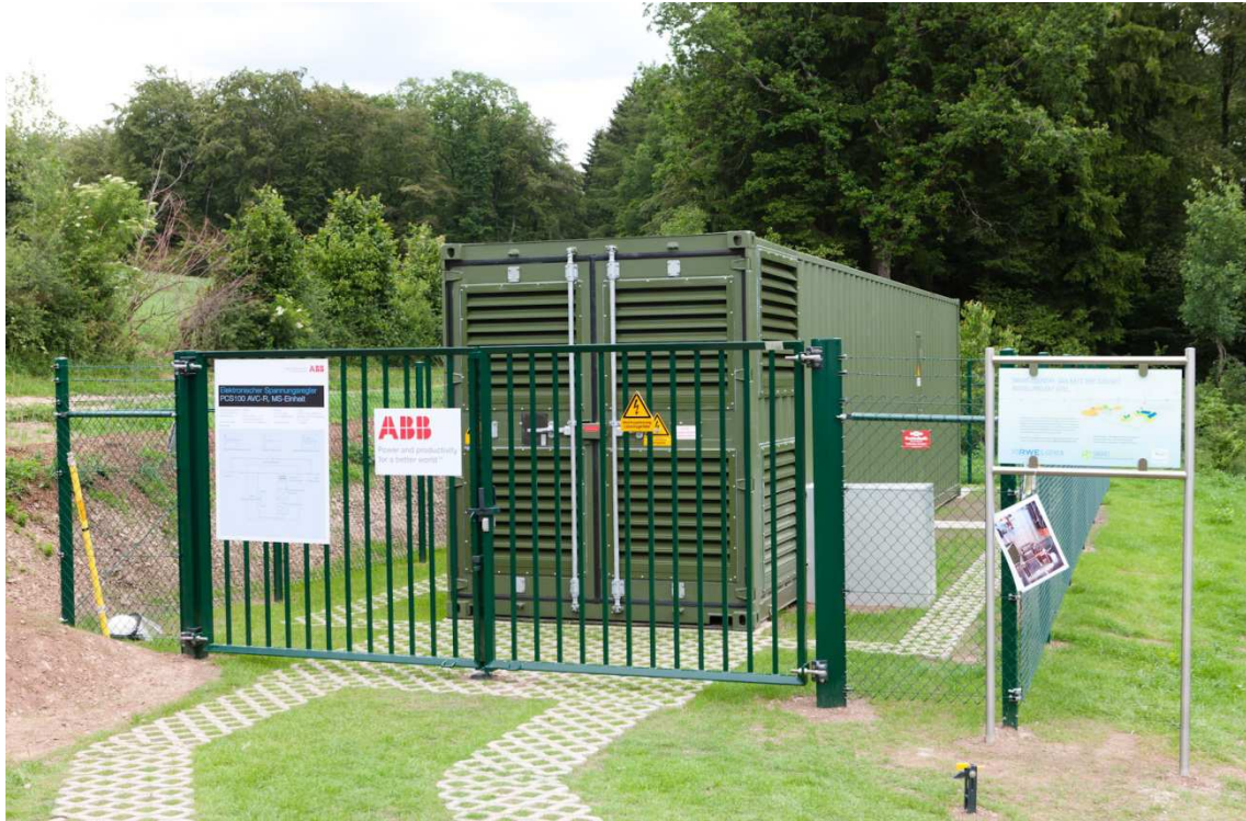
Figure 3-2 : PCS100 AVR (MV Level – Outdoor Installation)
