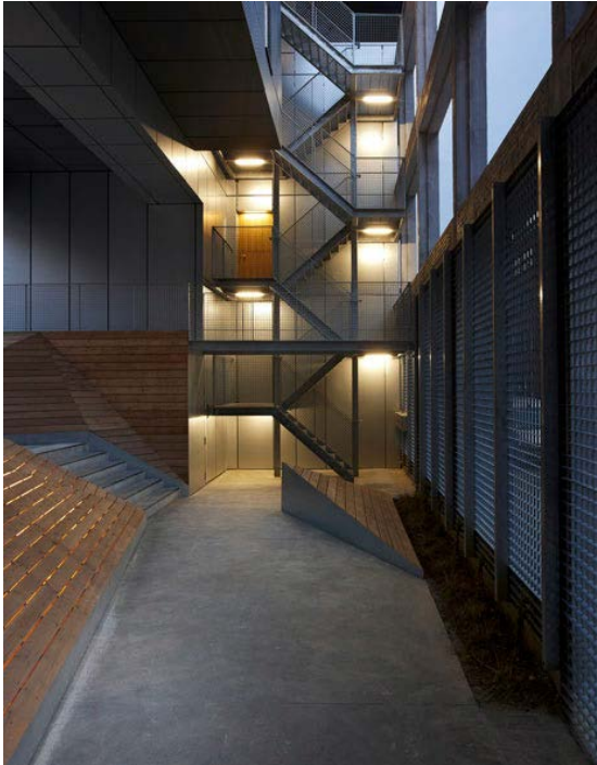
Figure 3.46: Le Lorrain. Hot dip galvanized steel mesh along the original scrap metal building street facade.
