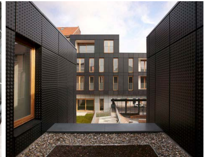
Figure 3.48: Le Lorrain. Dark grey metallic sheet cladding contrasted by wooden window frame.
