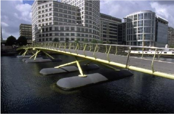
← Figure 2-10 West India Quay Footbridge, Anthony Hunt Associates (1996) London The bridge is steel structure supported by the splayed legs welded to circular plates that are bolted to the foam-filled pontoons above the water surface.
