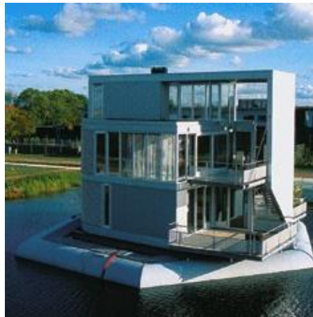
↑ Figure 2-7 Watervilla, Hertzbrger, H. (2002), Middelburg, Netherlands a floating house island that stands on a hexagonal pontoon Source: Architectuurstudio HH, http://www.ahh.nl/
