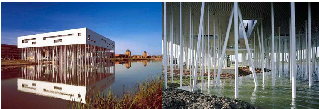
↑ Figure 2-15 Aluminium Forest, Haas, M. (1997-2001). Nouten, Netherlands a museum supported by aluminium tubes provided to offer load bearing function and house services Source: Flesche, F. Water house , (London: Prestel, 2005), pp. 26.
