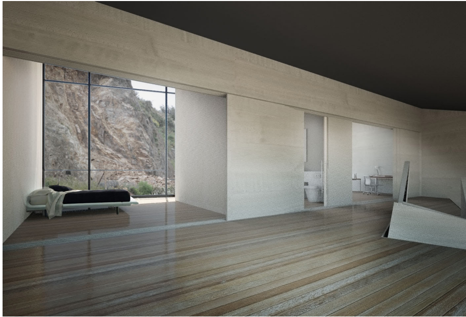
Figure 94: Interior render of mezzanine floor featuring sliding timber partitions to open up or close off the private areas (House 5) Walls exposed CLT white washed, flooring is White Oak - Author's own
