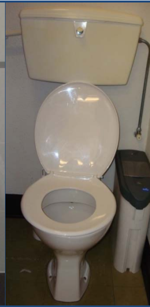
Figure 9.9: Single Flush Cistern Toilet
