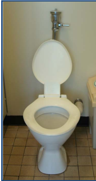
Figure 9.7: Flush Valve Toilet
