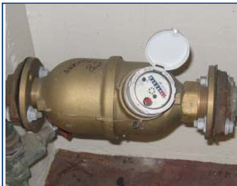
Figure 9.3: Main Water Meter
