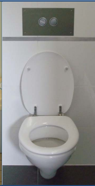
Figure 9.8: Dual Flush In-Line Toilet
