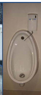
Figure 9.36: Leaking Urinal Solenoid
