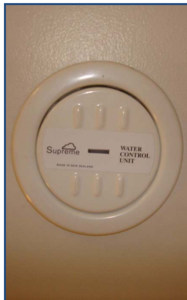
Figure 3.17: Motion Sensor for Urinal
