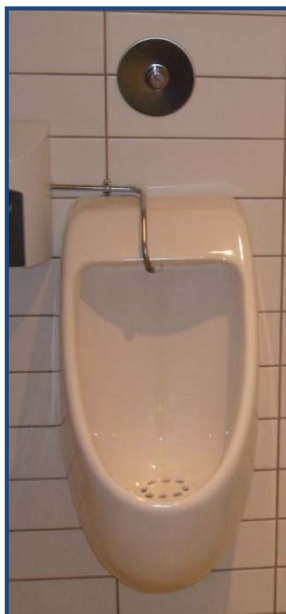
Figure 3.16: Manual Flush Wall-Pod Urinal
