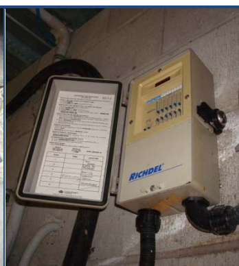
Figure 9.33: Irrigation Control Unit
