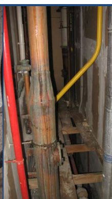
Figure 9.34: Leaking Pipe in Duct
