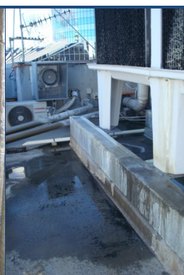
Figure 9.35: Heavy 'Splash' from a Cooling Tower
