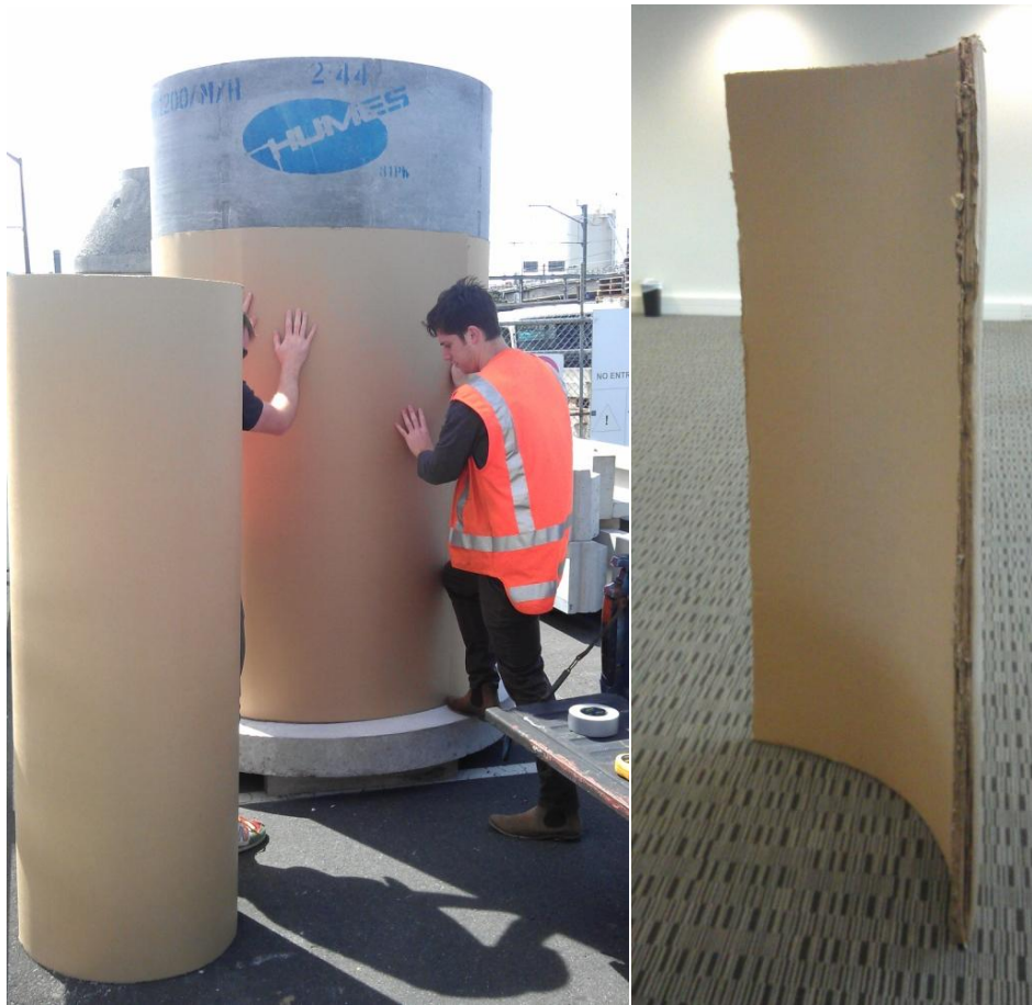
FIGURE 11: BENDING CARDBOARD AND THE FINISHED PANEL
