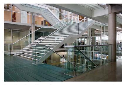
**Figure 6.11 Carre d'Arte stairs,** viewing across atrium. Glazing to stair treads, glazed balustrade, open nature of stair flights, all help maximize views in and across atrium. *Source: Villela.*
