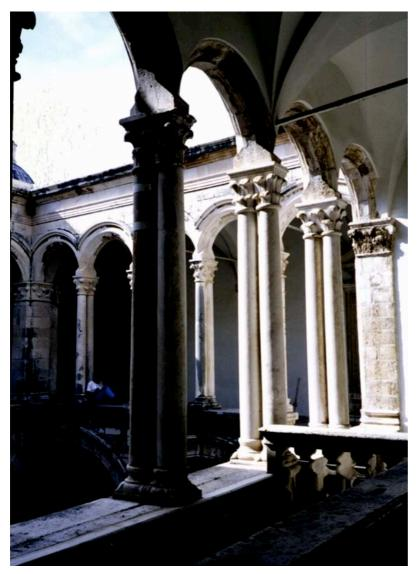
**Figure 5.1.12 Oblique view of upper colonnade**. Double columns add strength and lightness to the atrium facades, but also increase the amount of solid obstructions in the perforated façade. The balustrade to 'back of house' staircase is visible in lower right of photo. *Source: author (1998)*.
