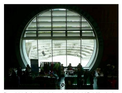
**Figure 5.3.8 Oculus,** viewing back over city, heavily shaded. The building takes the opposite viewpoint to light that Foster's media gallery at Nimes. Here, direct sunlight is banned, and daylight is actively avoided. *Source: author (2012).*
