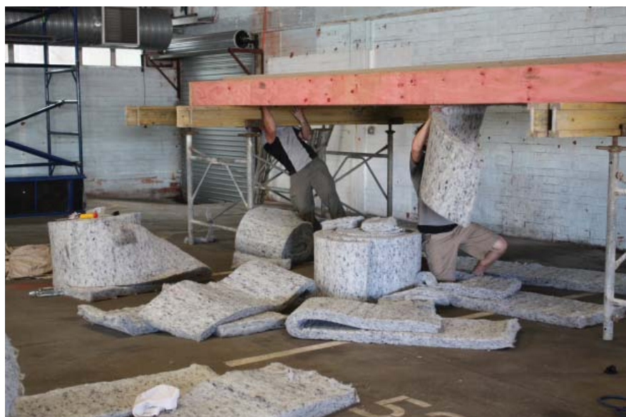
Figure 21: Installation of wool insulation
