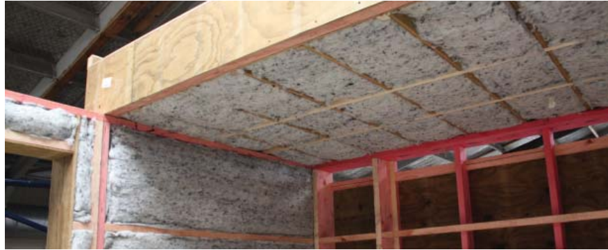
Figure 22: Installed wool insulation in roof and wall
