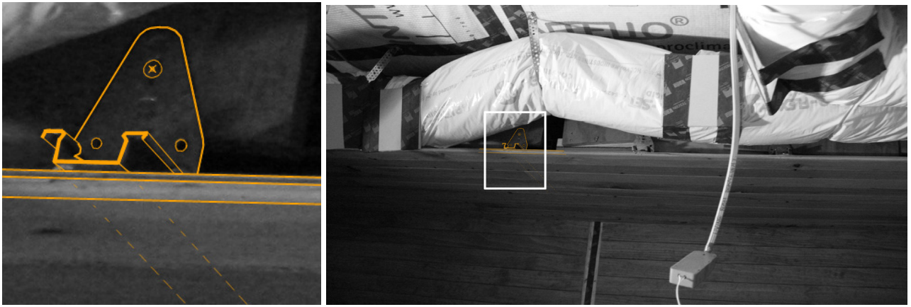
Figure 8.21 The use of the Rondo system to support the removable ceiling was trialled in the living room 'nook', the end of the bulkhead with fewer services. Instead of a solid rectangular duct, the engineering team specified a flexible duct for this area, so that plywood struts could be attached to the roof structure above. Rondo clips were fixed into the plywood.
