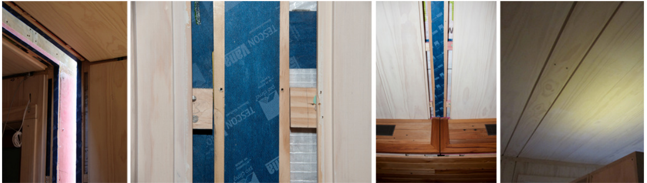
Figure 8.12 Photos during construction of (left – right): fixed panels either side of the module joint; the module joint taped at wall and ceiling to complete the airtightness envelope; and the finished ceiling lining at the module joint
