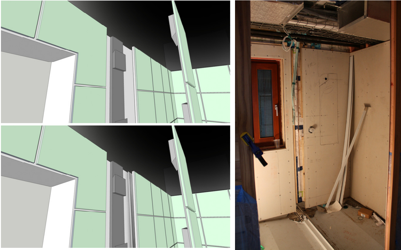
Figure 9.9 A full height flashing slots behind permanent lining on either side of the module join (left) and (right) photo of the bathroom after installation of stainless steel shower trays. The full height flashings and the cap flashing can be seen leaning against the wall in the corner.
