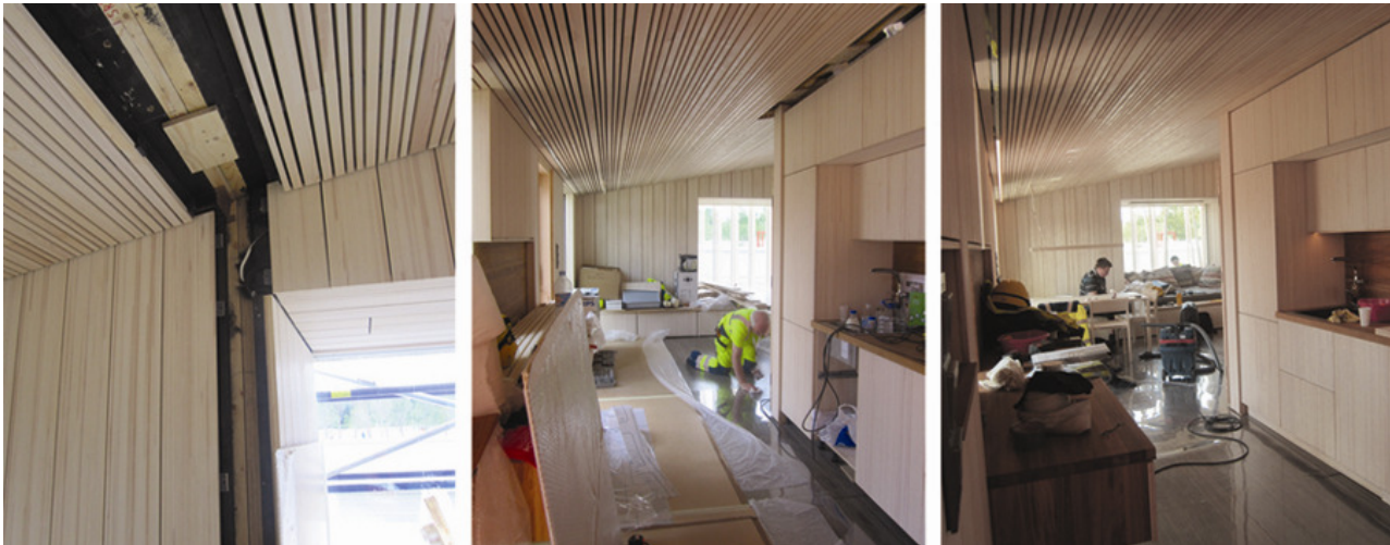
Figure 8.7 Finland's 2010 European Solar Decathlon house showing the interior timber finish in line with the module join
