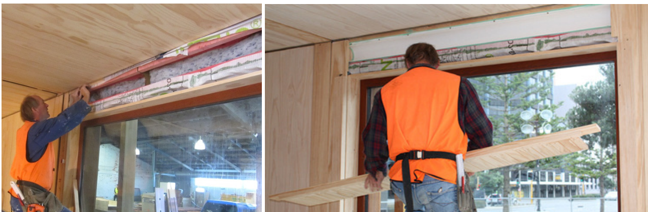
Figure 9.4 (left) The airtightness membrane was reopened and some of the insulation removed to accommodate the blind within the wall. The gusset plate at mid span can be seen notched. (right) the guttering profile was fixed into the cavity, and sealed with [green] adhesive to ensure airtightness. The lining panel was then fixed over this to await blind installation at a later date.
