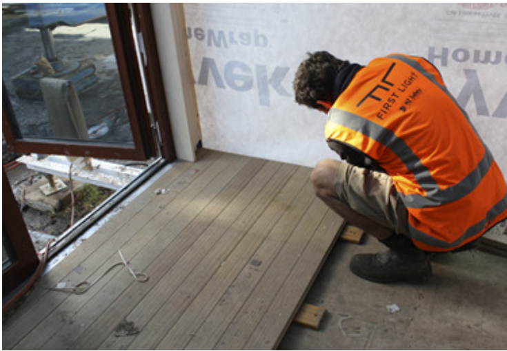
Figure 9.13 Decking panels being removed during disassembly of M3
