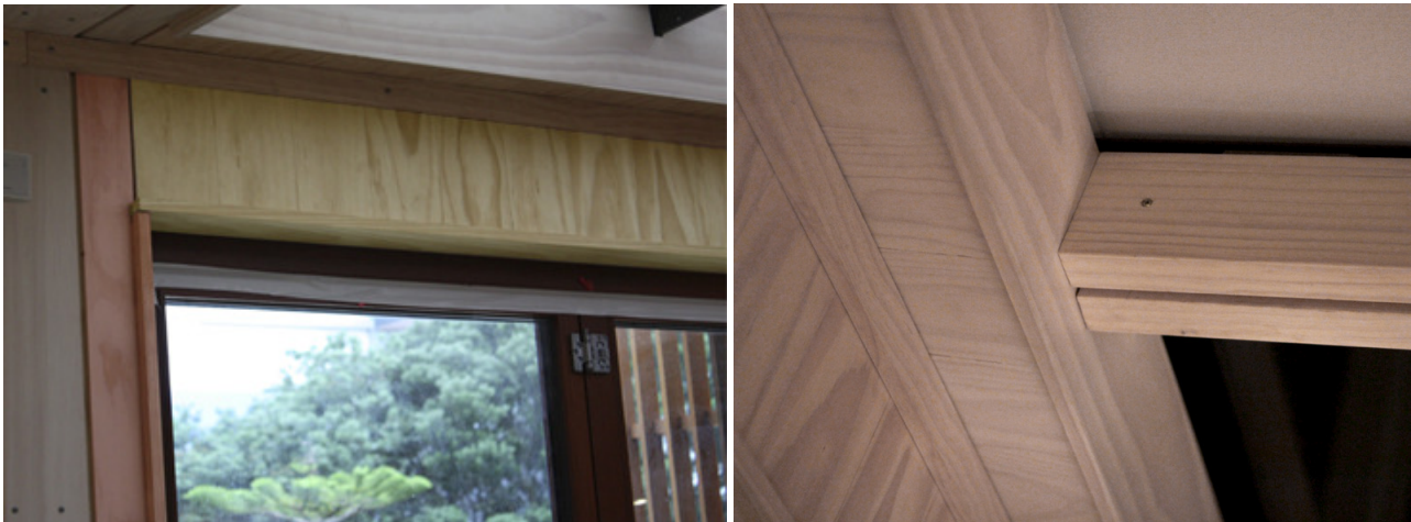
Figure 9.17 (left) L-shaped lining panels on the south side of M3 are simultaneously door head (yellow) and reveal (red) and (right) the L-shaped panel, detailed the same, as the skylight reveal
