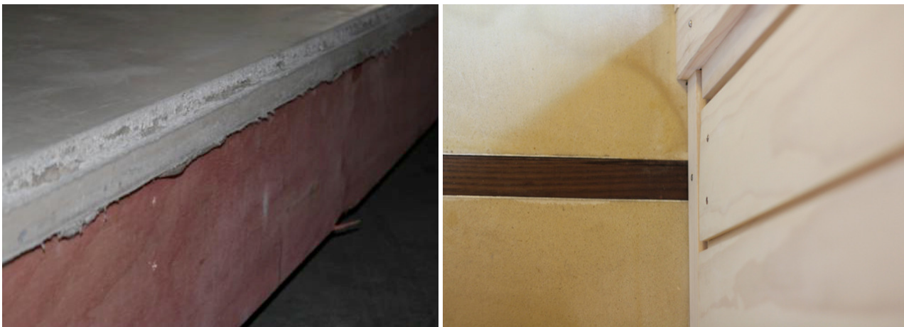
Figure 8.23 The module edge that arrived on site (left) and the finished floor join after a long process of remediation (right)
