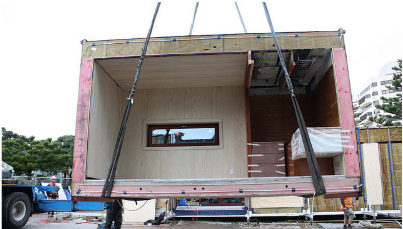
Figure 3.1 Lifting of the first module in Wellington; emphasising the need for care of edges and pre-installed furniture PHOTO CREDIT PAUL HILLIER
