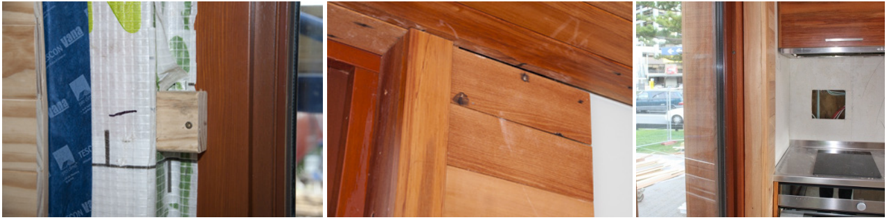
Figure 9.16 Northern [kitchen] M3 wall section without lining (left) and (right) with L-shaped lining/reveal component attached
