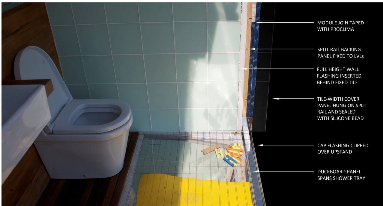
Figure 9.10 An overview of the bathroom finishing sequence
