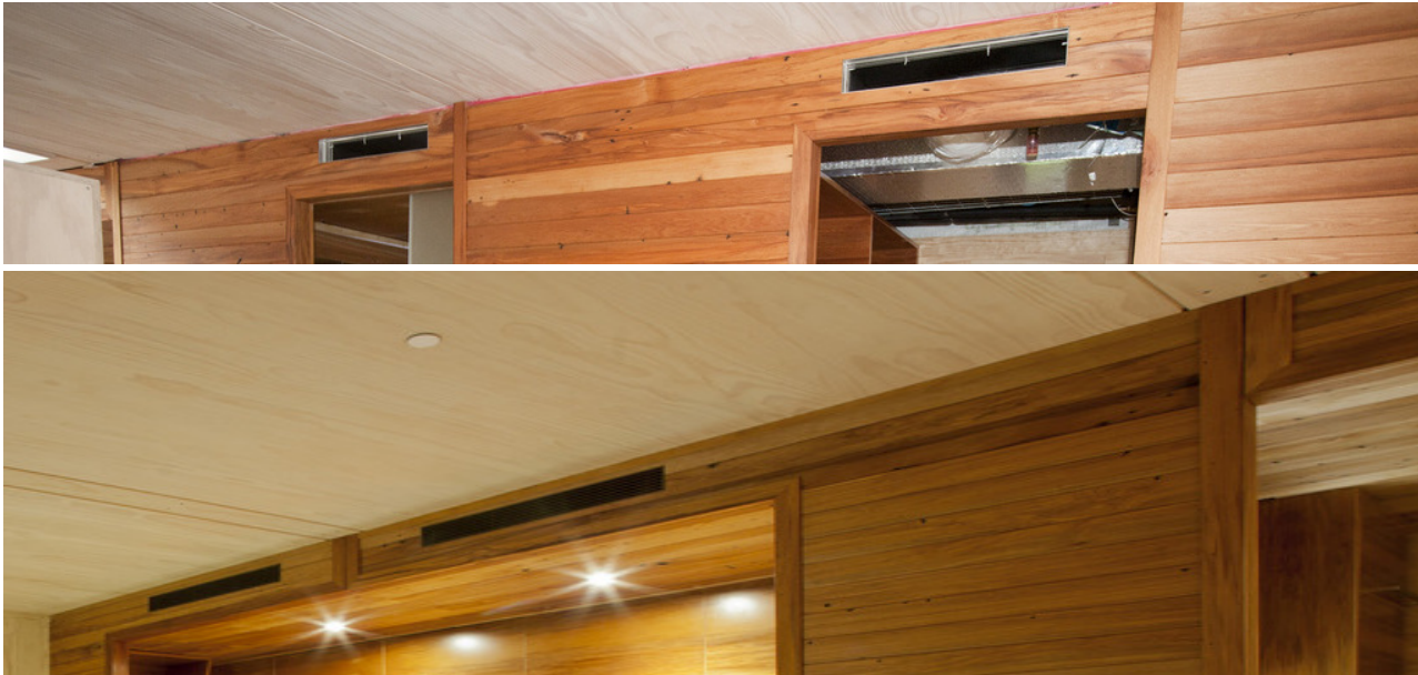
Figure 8.16 Treatment of the module junctions on the services core wall – modules 4, 5 and 6 during construction (above) and modules 1, 2 and 3 finished (below)
