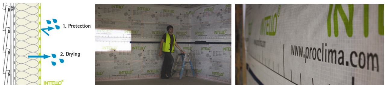
Figure 8.5 Proclima Intello vapour release membrane: properties (left) and (right) VRM applied to the internal walls of the living room IMAGE CREDIT (left) PROCLIMA NZ
