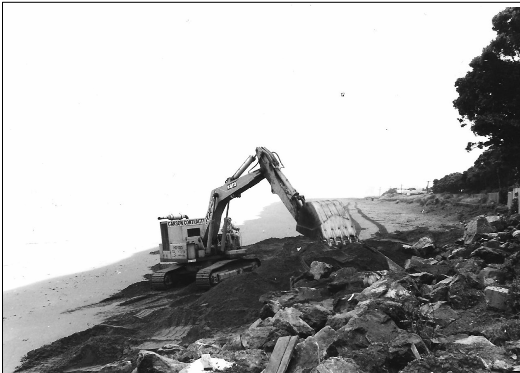
Figure 3.10: Construction of the boulder rip-rap in northern Robinson Bay in response to erosion in the 1960s and 1970s (Courtesy of the Eastbourne Historical Society).
