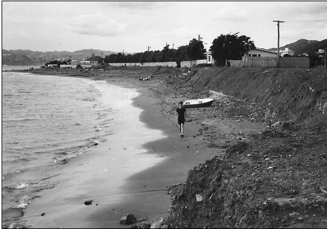
Figure 1.1: Erosion at the H.W. Shortt Recreation Ground, northern Robinson Bay, Eastbourne following the stormy period of 1968 that included the Cyclone Gisele on April 10 (Cunningham, 1969, courtesy of the Eastbourne Historical Society).
