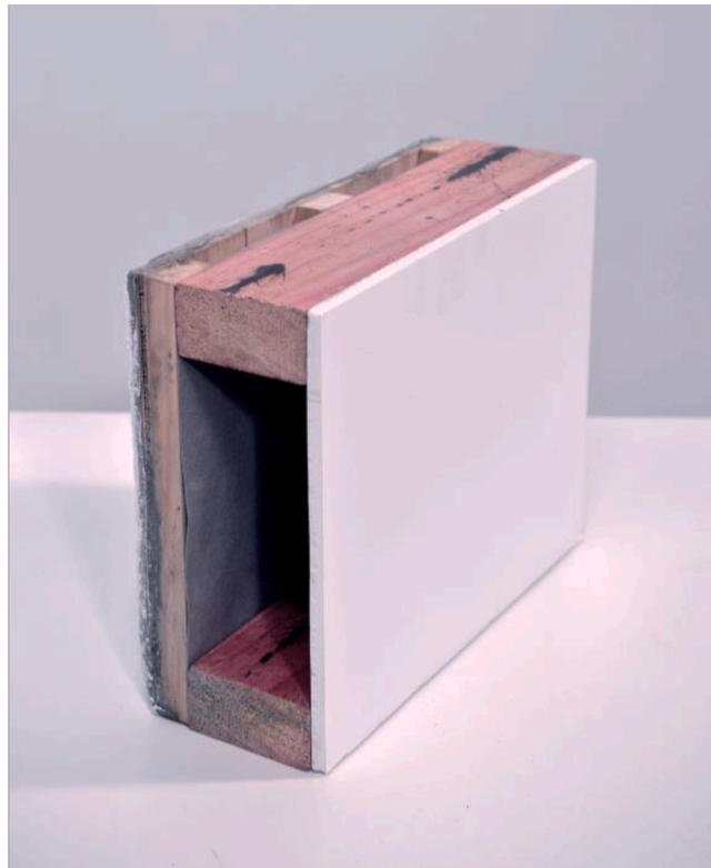
Fig. 2. Technical cross-section drawing of platform timber framing in New Zealand (left) and a built section of that framing (right).
