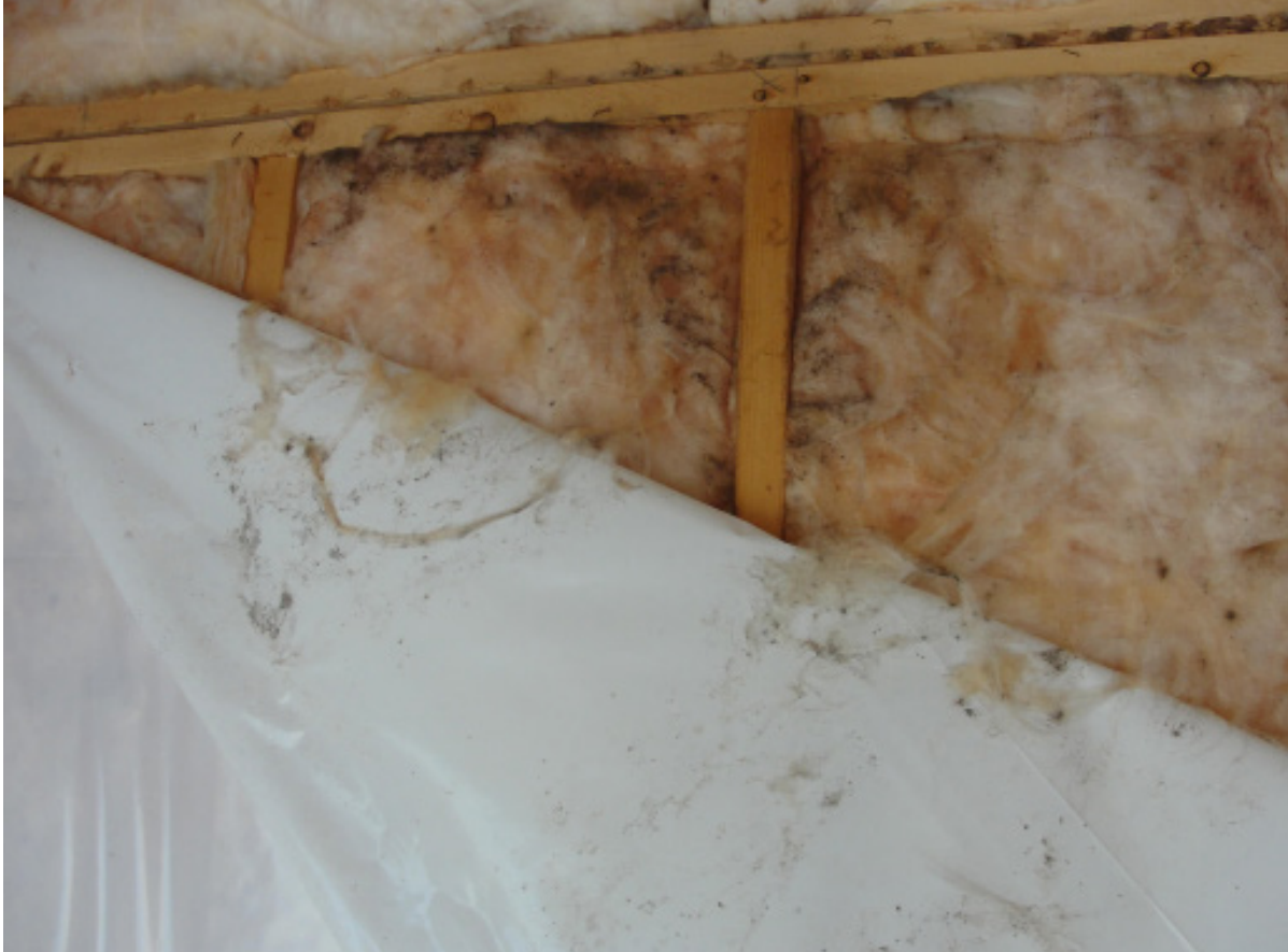
Figure 1.2. Mould in a timber framed building envelope on the building wrap and cavity insulation. Saltzman, 2012.
