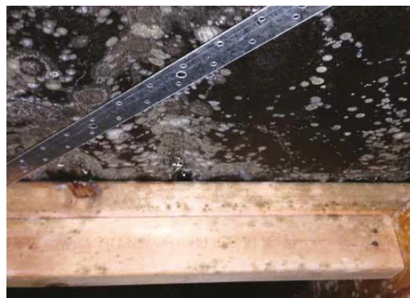
Figure 2.10. Mould growing on roof framing timber and roofing underlay in a vented roof in an Auckland house. BRANZ Facts Roof Ventilation #1: Roof Space Ventilation in New Zealand houses (p.1), BRANZ, 2018.
