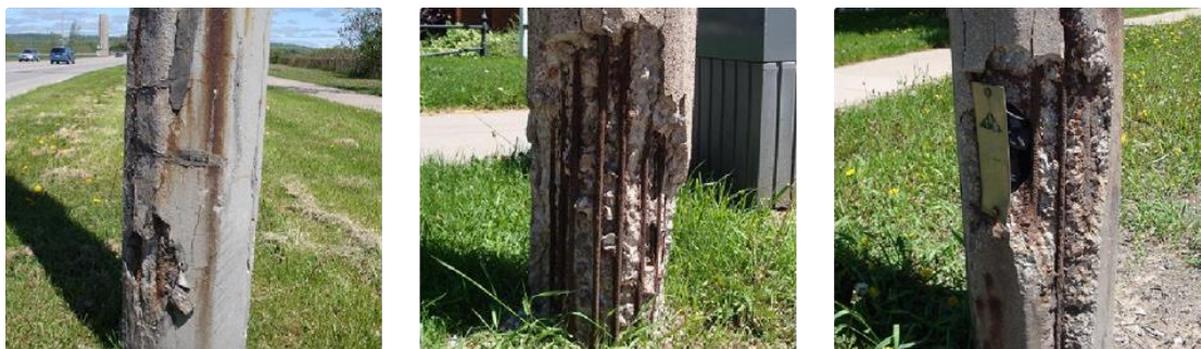
Figure 1 Examples of spalling concrete power poles where the corrosion has expanded and caused the concrete to crack and fall off making a clear visual sign of an issue.[2]
