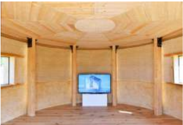
Note. The Gaia House, built in October 2018, has a 3D-printed outer shell made from a mixture of soil and other biodegradable materials such as chopped rice husks. The house is 30m2 and uses timber columns as structure to hold up the timber roof.10/2018
