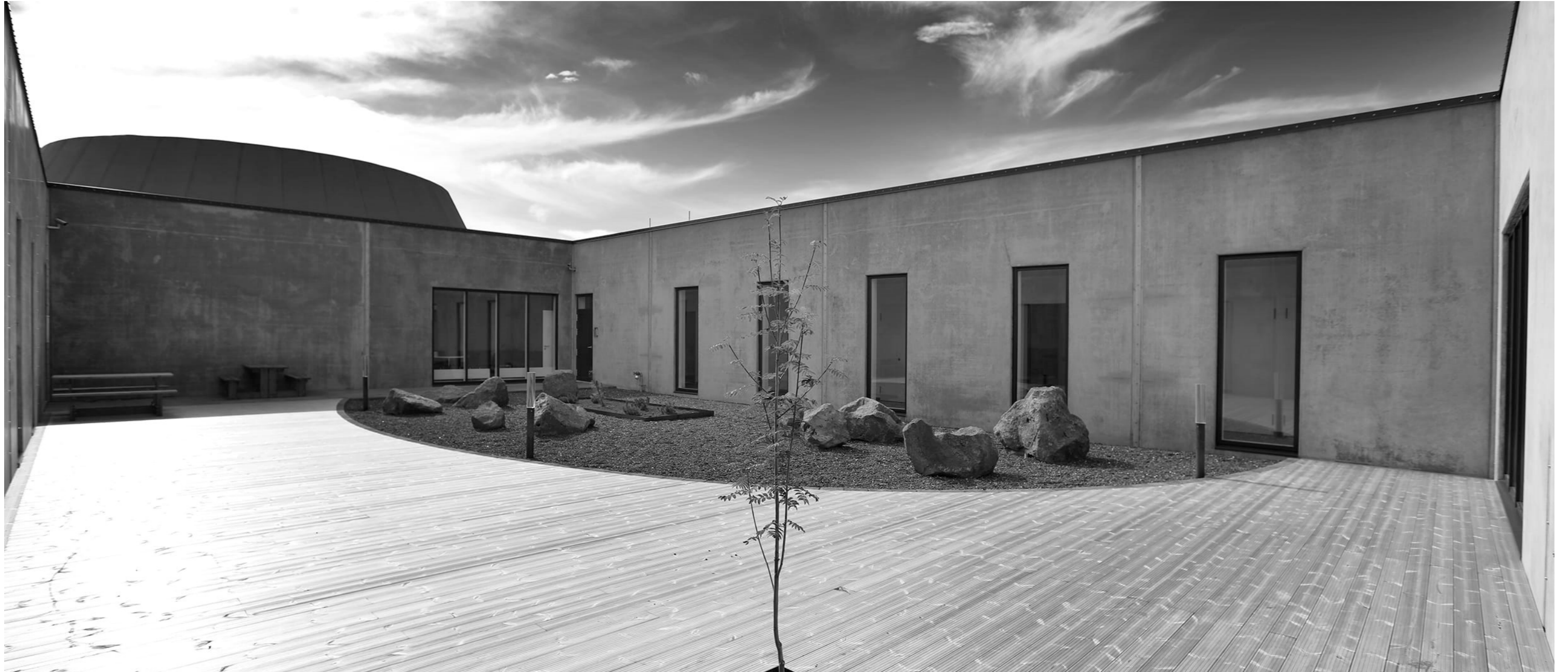
Figure 3.20 Holmsheidi interior courtyard
