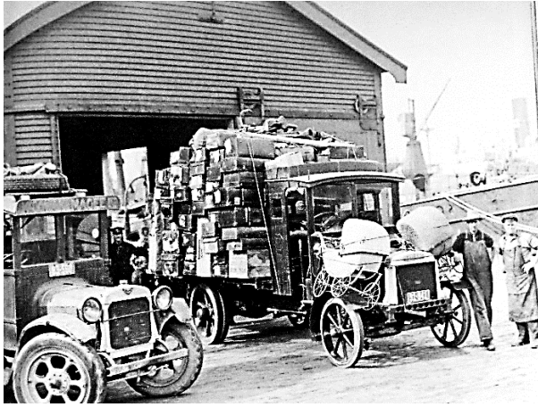
FIGURE 41: TRUCKS, WELLINGTON WHARF
