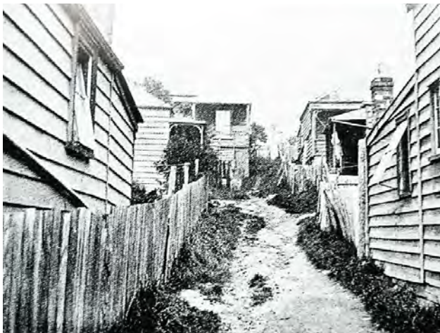
FIGURE 45 (ABOVE): POOR QUALITY HOUSING
